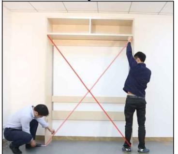
If the left and right gap size uneven, please check the diagonal size of bed frame first, if the diagonal size is right, please adjust the screw clockwise of the smaller gap side, back and forth debugging to the best of the situation
